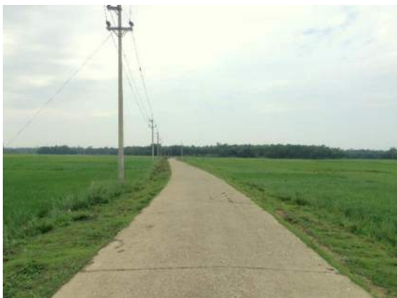
Figure 8.1: Submergible roads in the Surma haor system area
