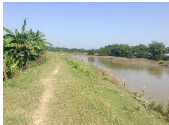
Figure 8.2: River bank embankment in the Surma haor system
