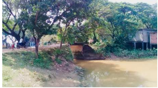
Figure 2.4: Box Culvert (1V) in Kalinagar
