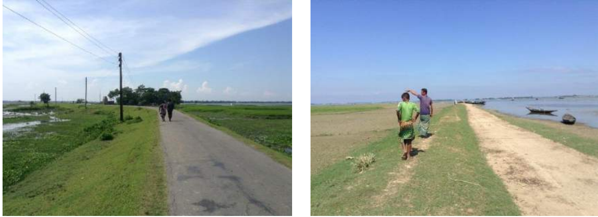
Figure 8.1: A submergible road and an embankment road that also used as the means of communication in Kalikota Haor, Sunamganj
