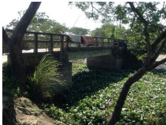
Figure 2.2: Narrowing the Width of the River by Constructing Bridge near Ramerpuri Beel
