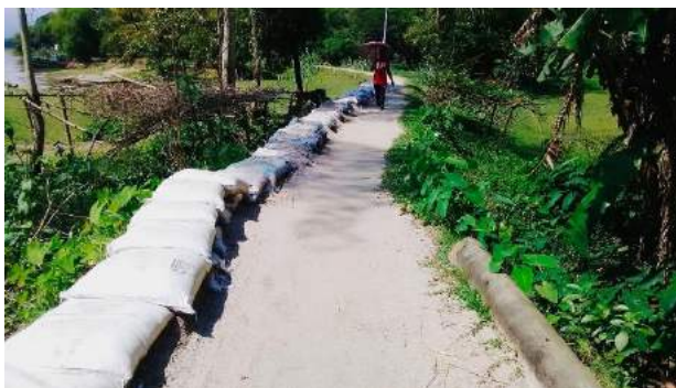
Figure 2.1: Dauki River Bank Protection
