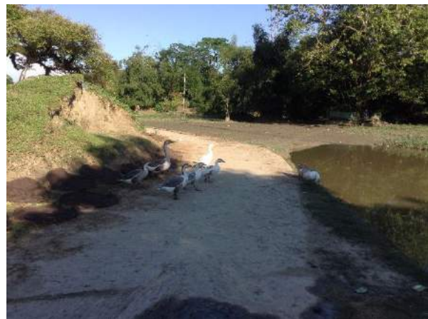
Figure 8.2: Submergible Road in the Study Area
